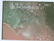
Photo: 723b, Tape/Media No.: T.O.S. 143, 08:58:32 47FT, Material Change, VCP Vitrified Clay Pipe FROM ABS
