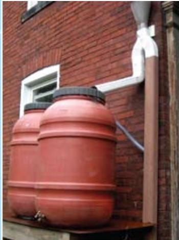
**Rain barrels or cisterns** collect and store water for later use in landscape irrigation. They can be purchased from a variety of outlets or they can be homemade. It is important that they are made of sturdy materials, have a cover that is difficult to remove and include an overflow system.
